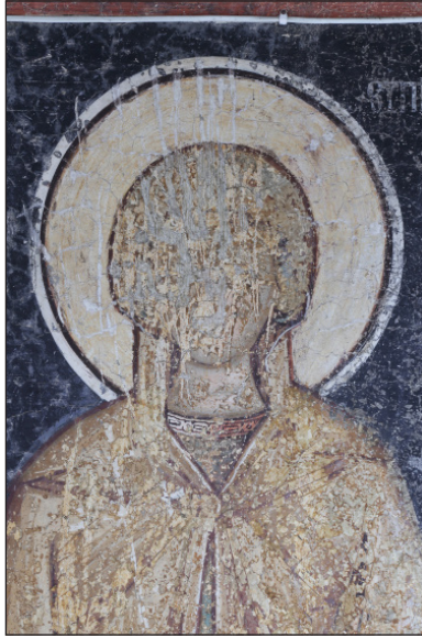
Figure 2: The exterior wall of Surpatele Monastery church, North Oltenia. Photo taken by Șerban Bonciocat
